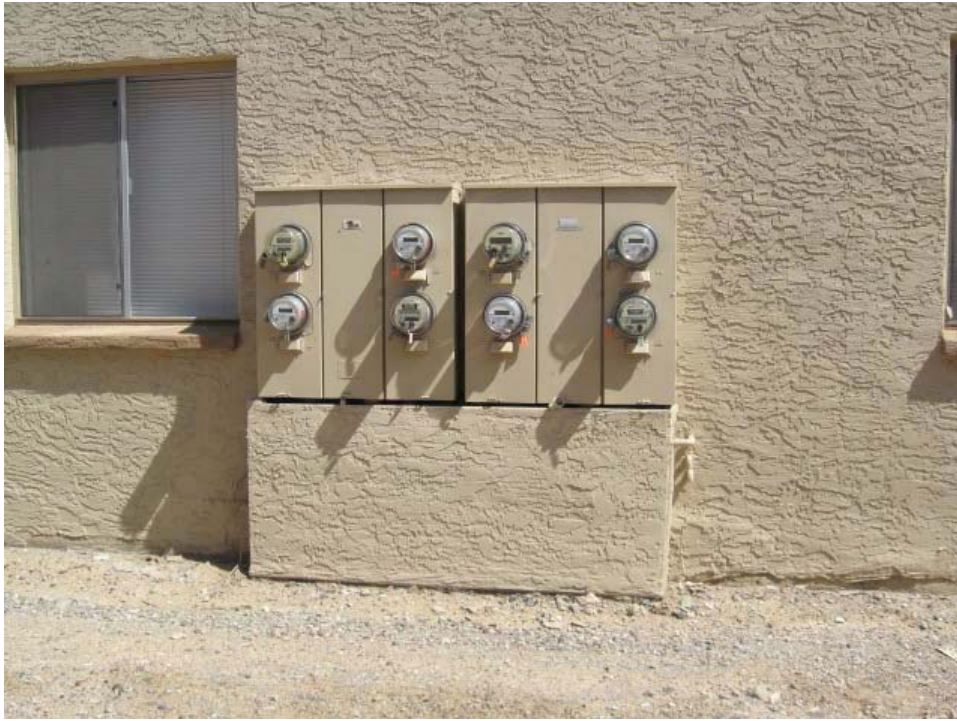
Typical Electrical Meter Section
