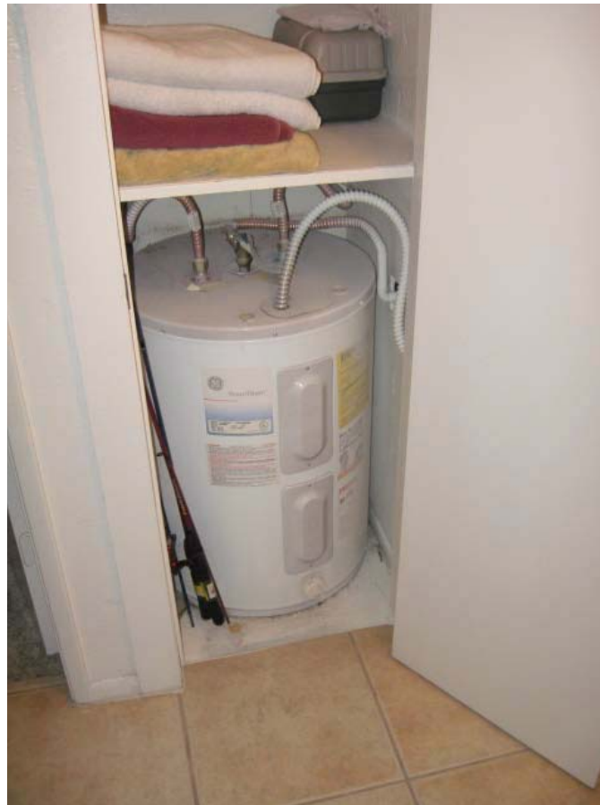
Typical Apartment Water Heater
